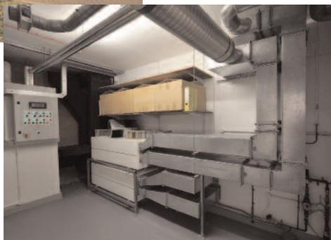
ilation. One of three ventilation levels is automatically selected according to PIR and timer controls. Unoccupied rooms are run at level one with no artificial lighting. Rooms in use are run at level two to provide adequate fresh air, with lighting if required. Level 3 is
